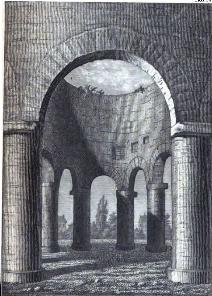
ANCIENT STRUCTURE IN NEWPORT, RHODE-ISLAND, THE VINLAND OF THE SCANDINAVIANS.
